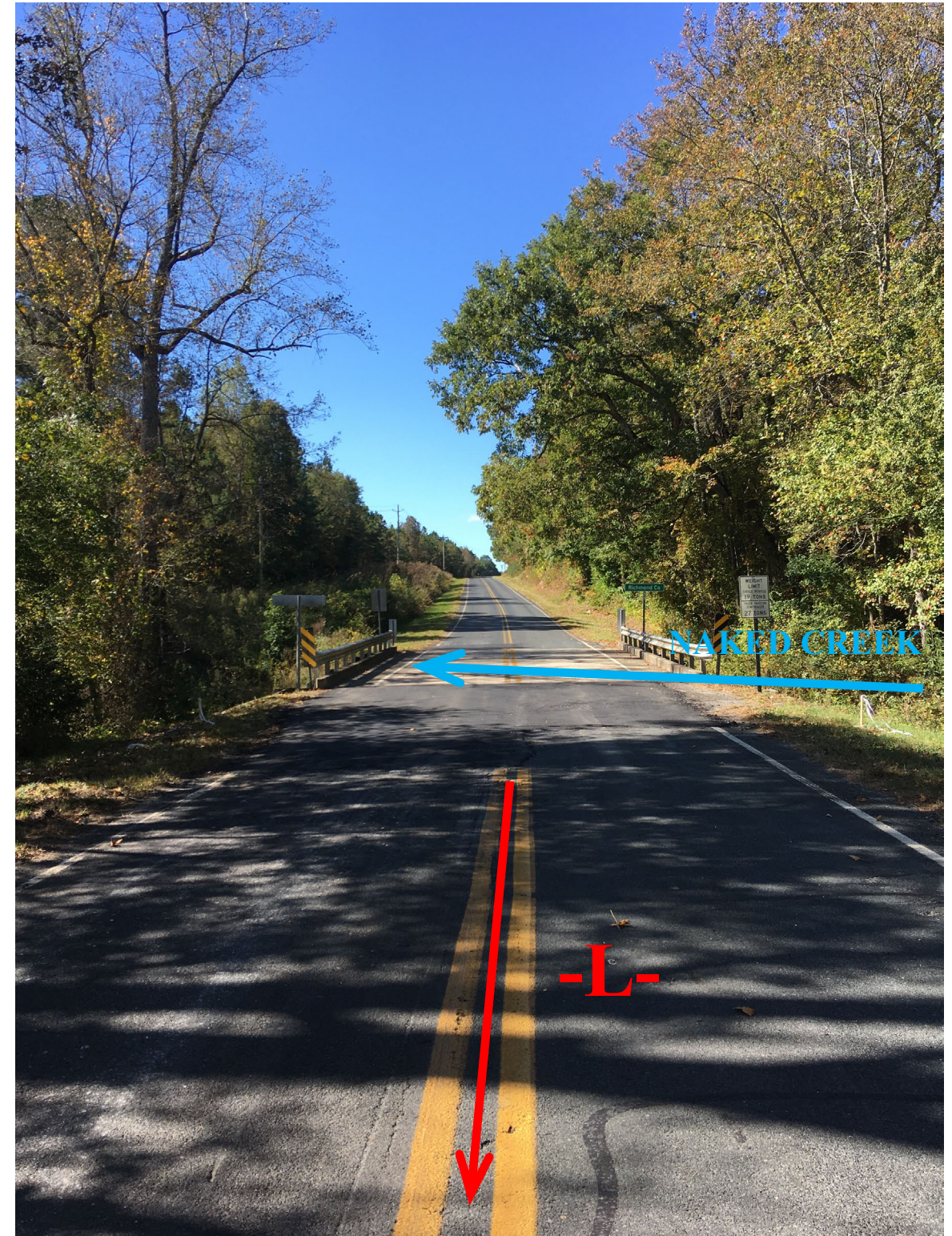
Looking West towards End Bent 2
