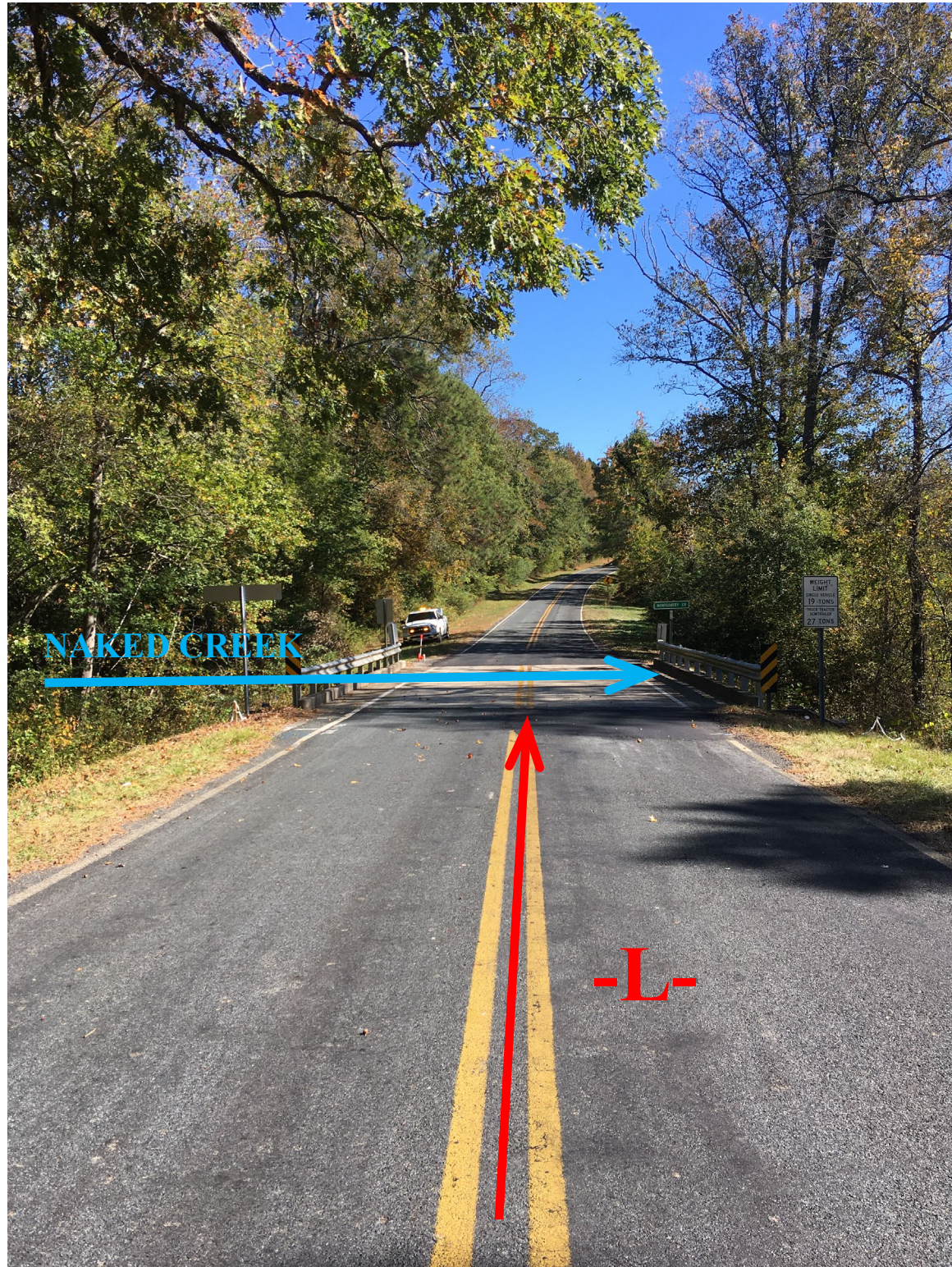
Looking East towards End Bent 1
